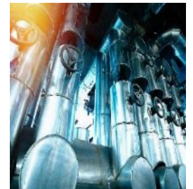
Cooling in Energy production 4 kW at -60C
